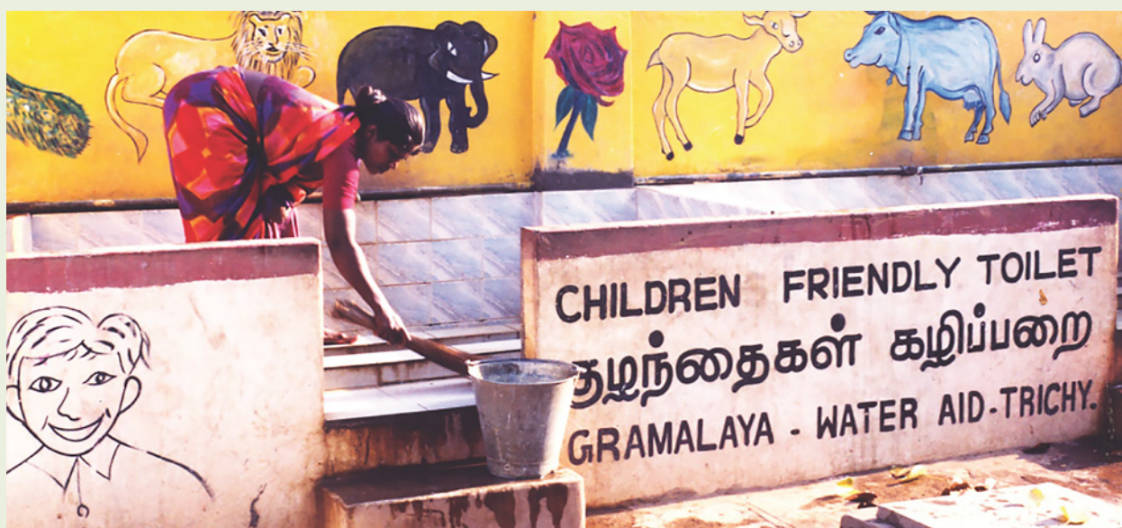
SHGs in Tiruchirappalli engaged in operations and maintenance of toilet
